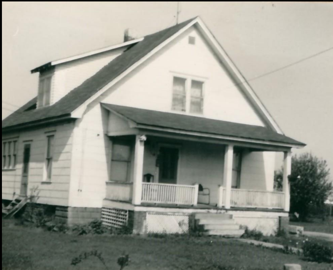
North Elm Street
